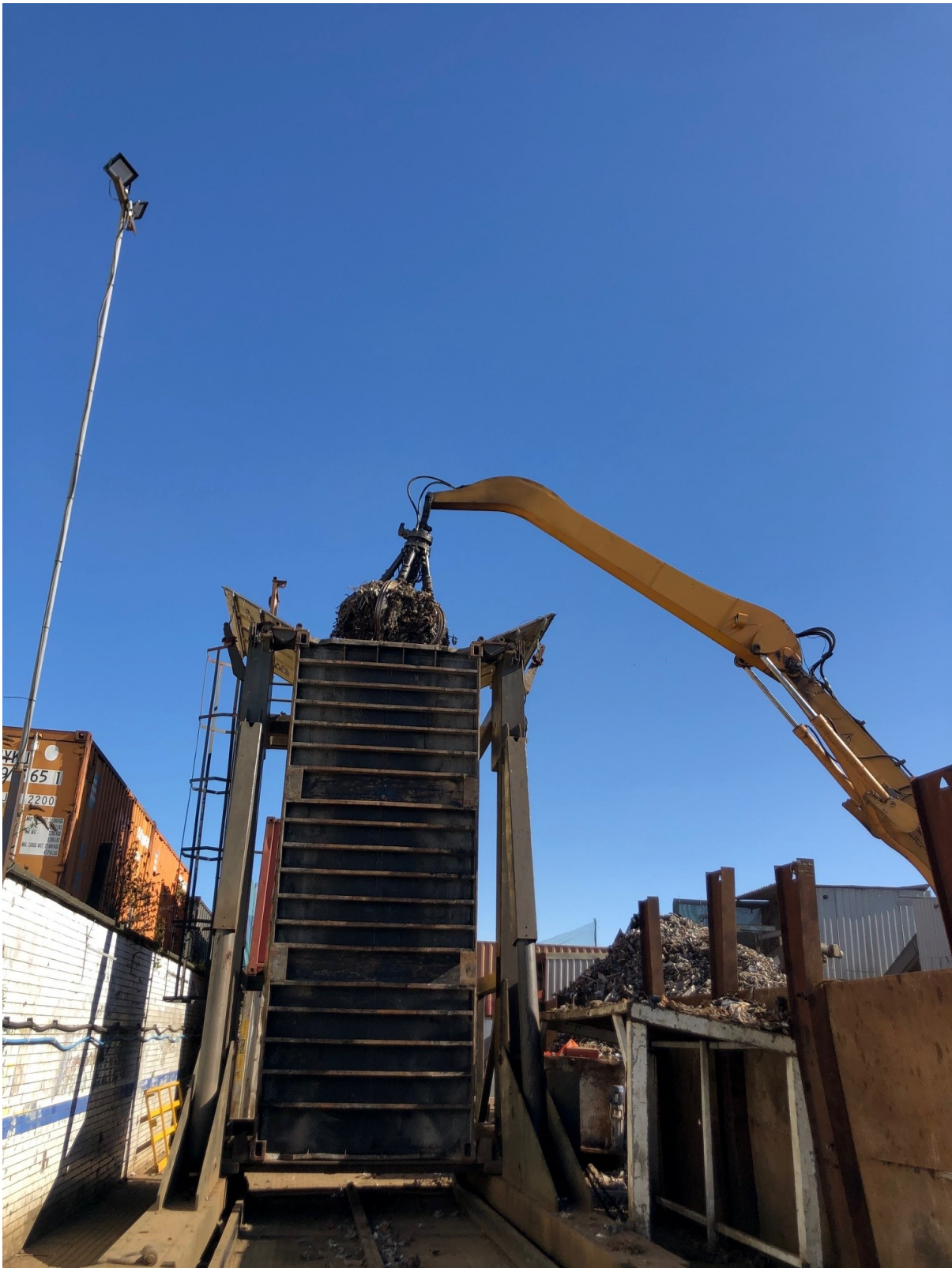
Photo 4 – Container Inverter and Crane Claw
